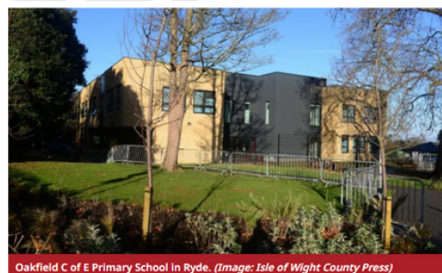
Oakfield C of E Primary School in Ryde. (Image: Isle of Wight County Press)
